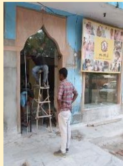
Construction in progress
